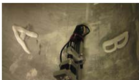
Fig.15 Inside of the measured pipe
